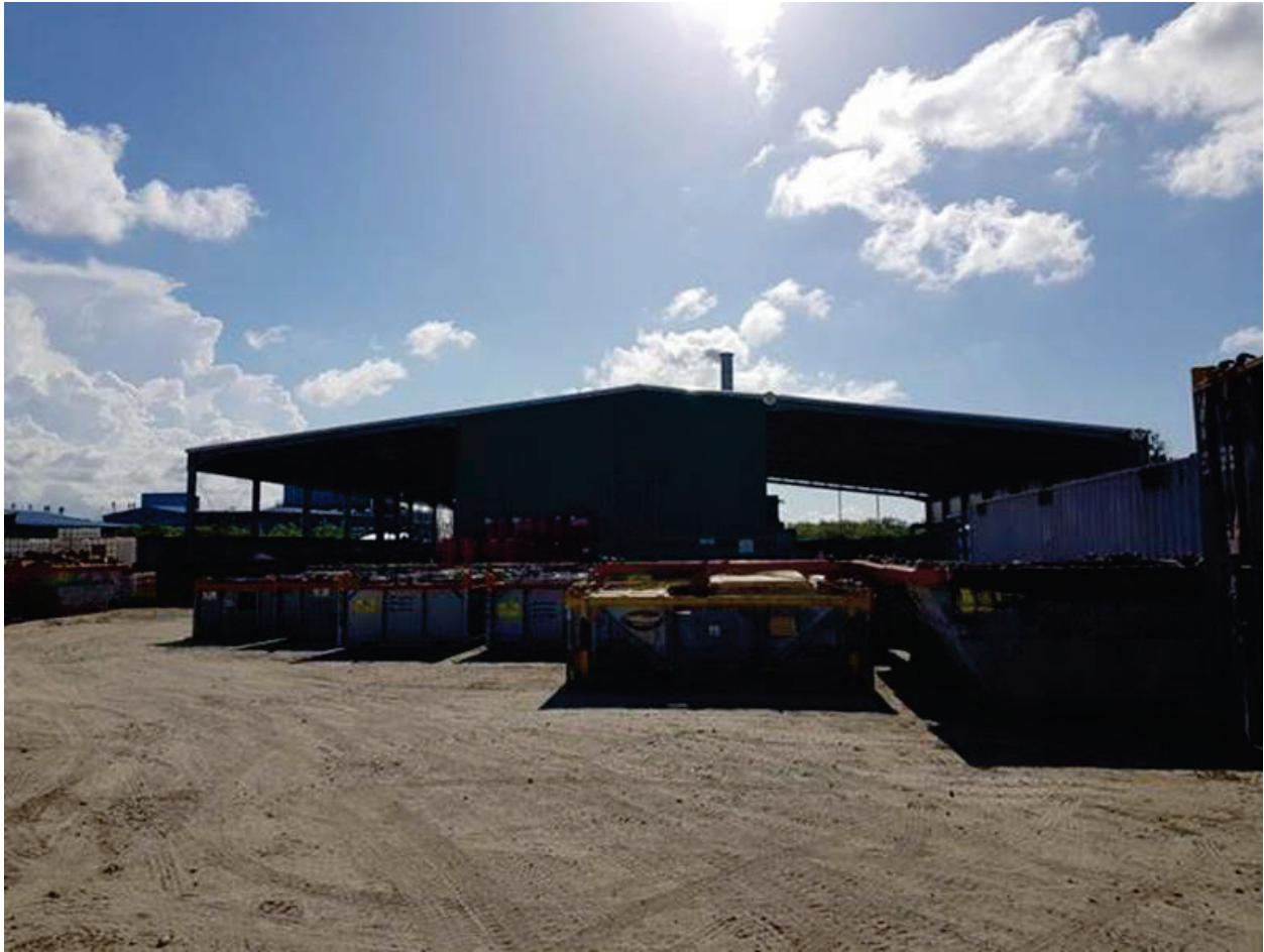
Figure 2.10-5: Typical Waste Management Facilities at Shorebase
