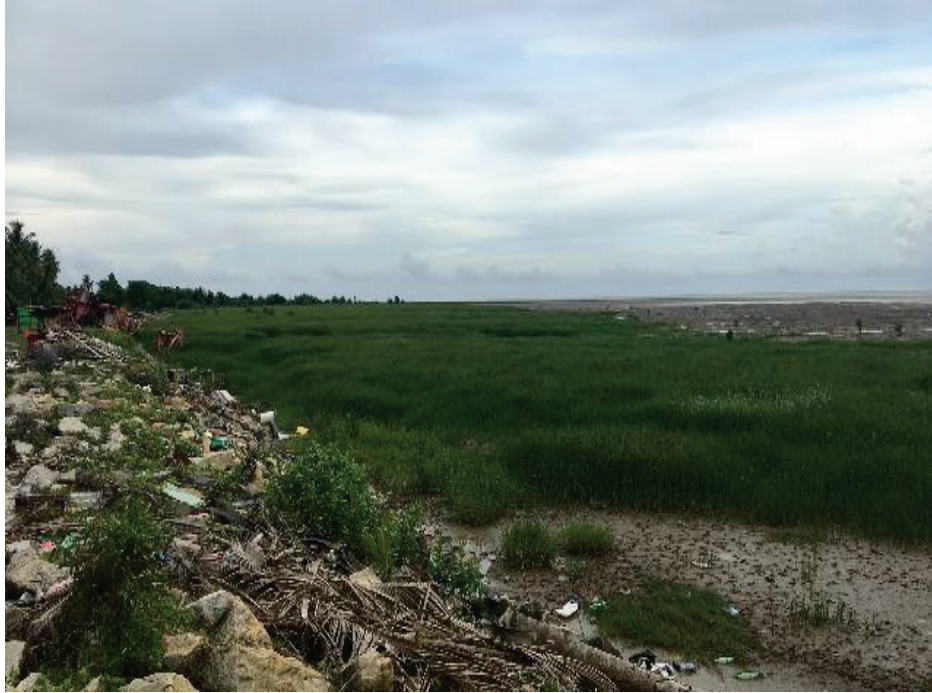
Figure 7.2-11: Saltmarsh Habitat in Region 2 that Developed after the Installation of a Groin
