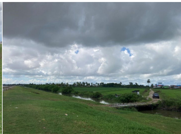
Seawall with pedestrian bridge
