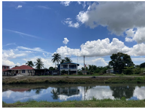
North side of Canal 1
