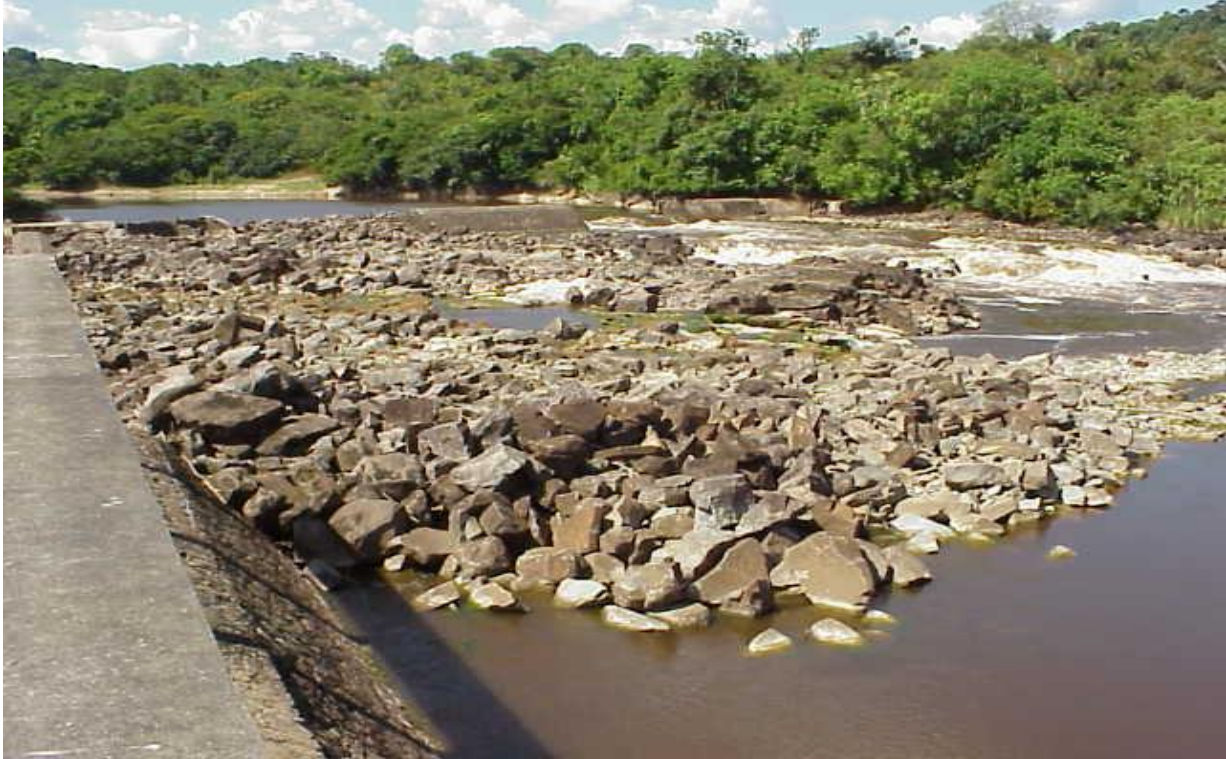
Damaged Section (left top) and Sluce Aperture Section (right top) of Spillway Weir
