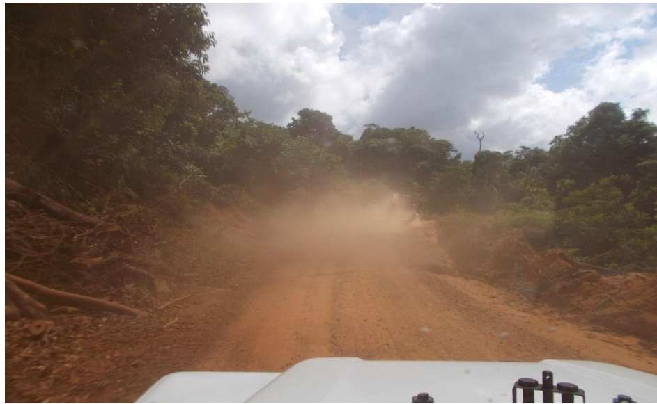
Figure f: Example of dust nuisance along the Kartabu –Puruni Road
