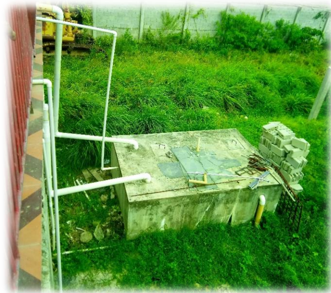
Figure 7: Septic tank situated south of the hotel
