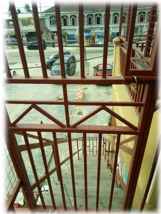
Figure 10: Northwestern fire escape
