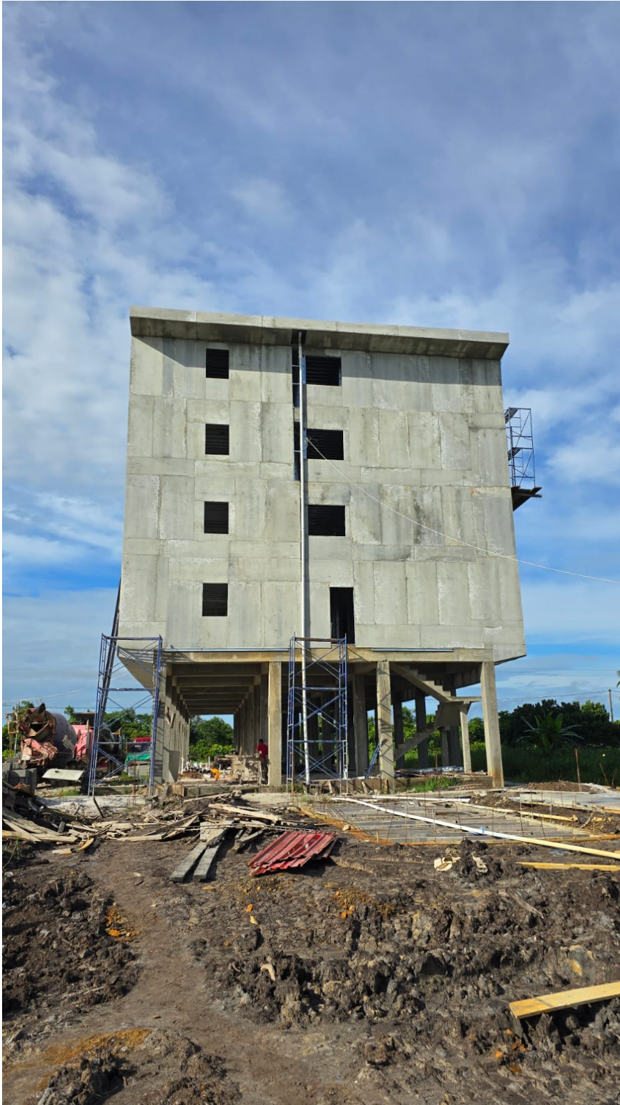
<Figure 18: Unfinished Rear View of Erected Hotel Building>
