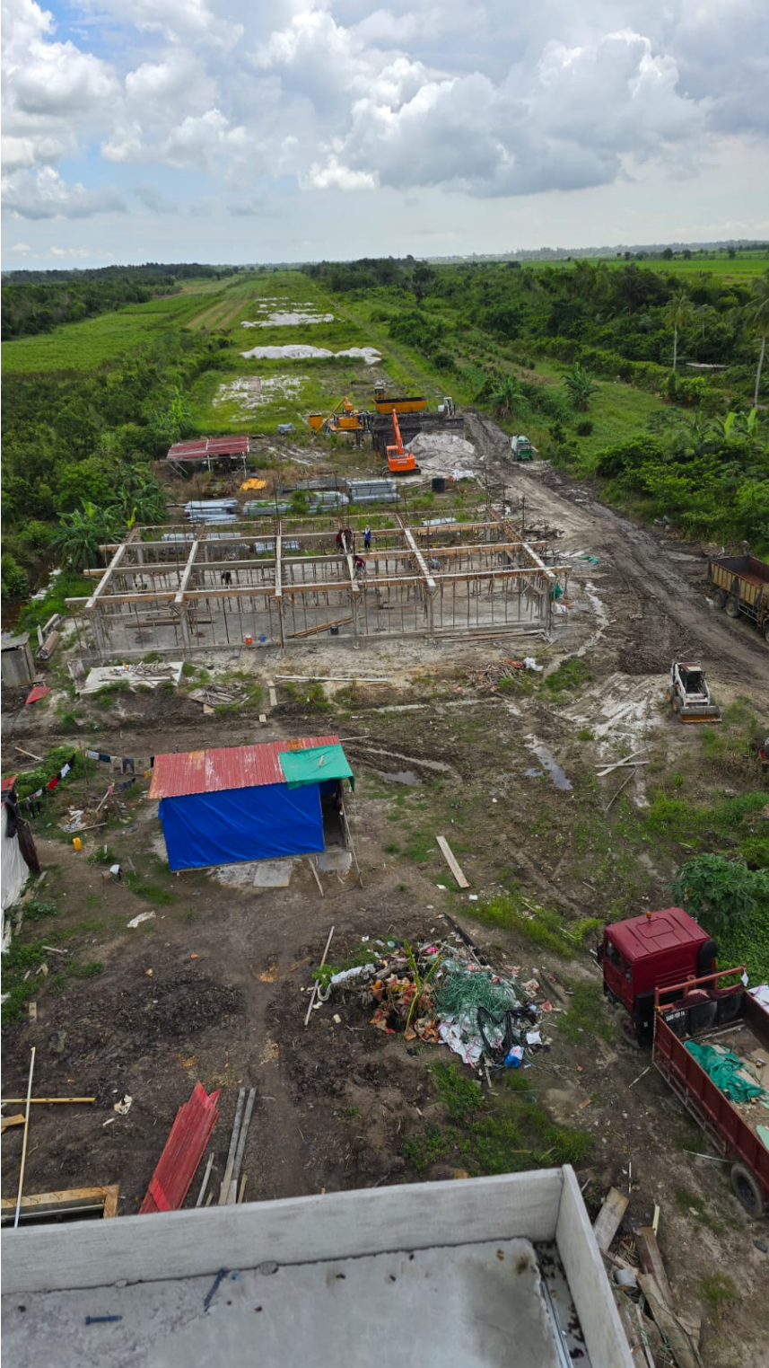
<Figure 19: Area Abck of Erected Hotel Building>
