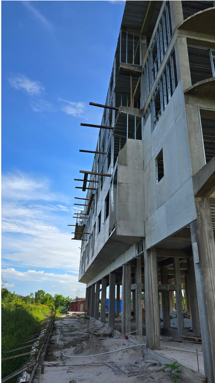
<Figure 17: Side View of Erected Hotel Building>
