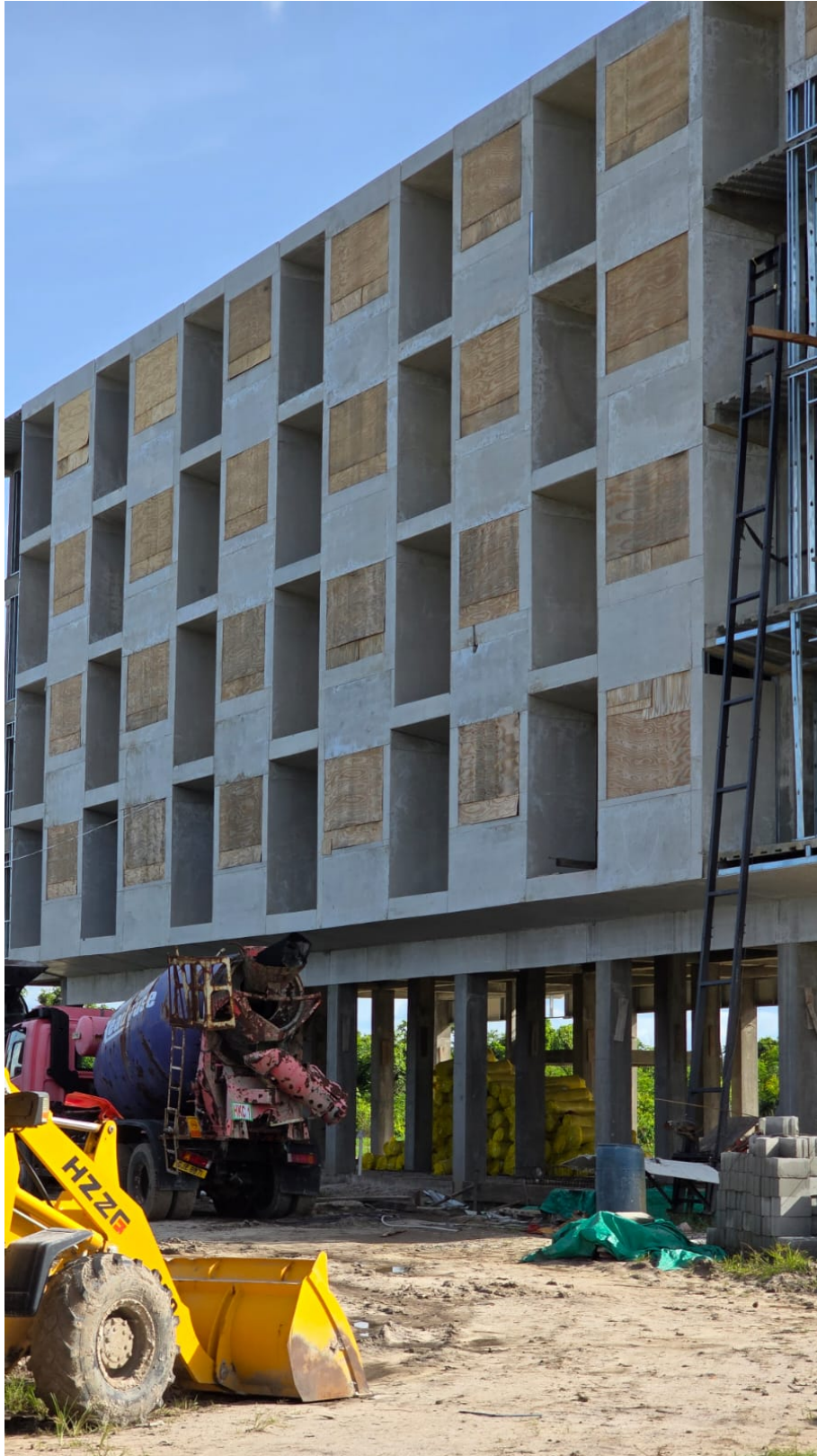
<Figure 16: Side View of Erected Hotel Building>
