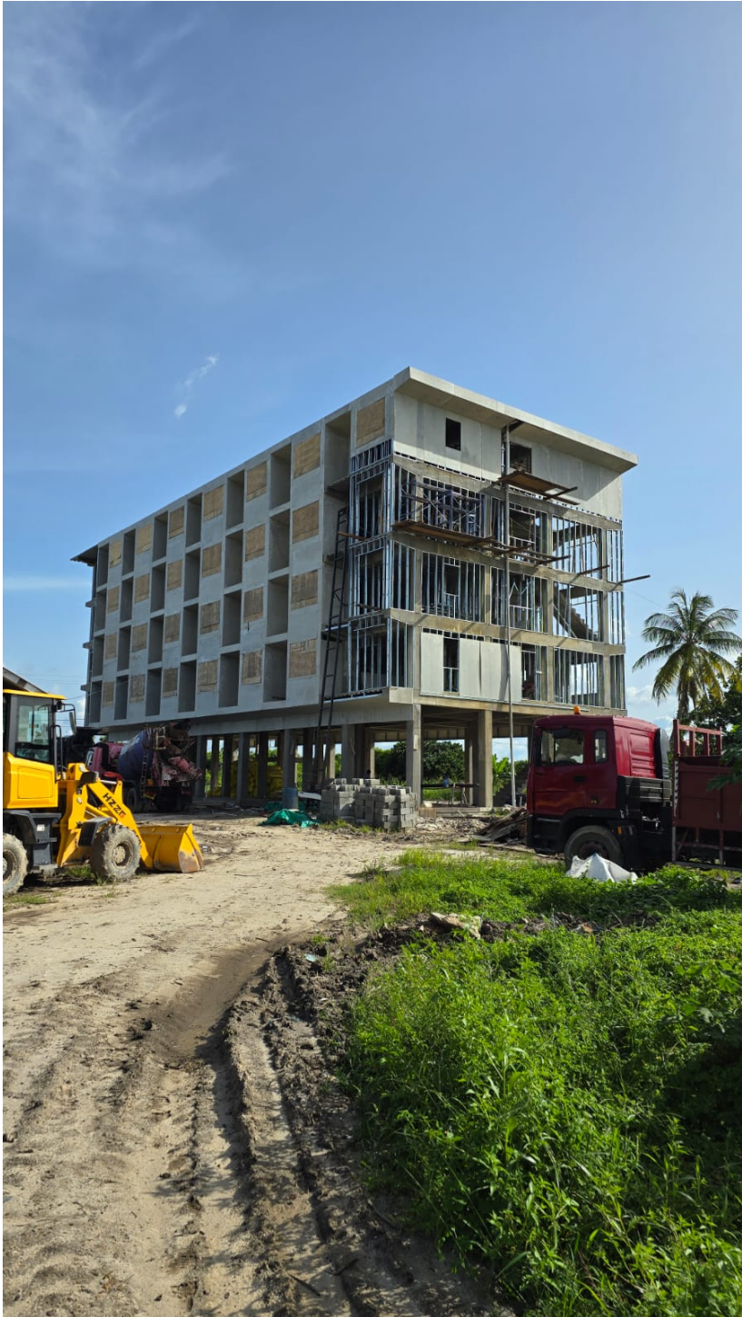
<Figure 14: View of Hotel Building being Erected>
