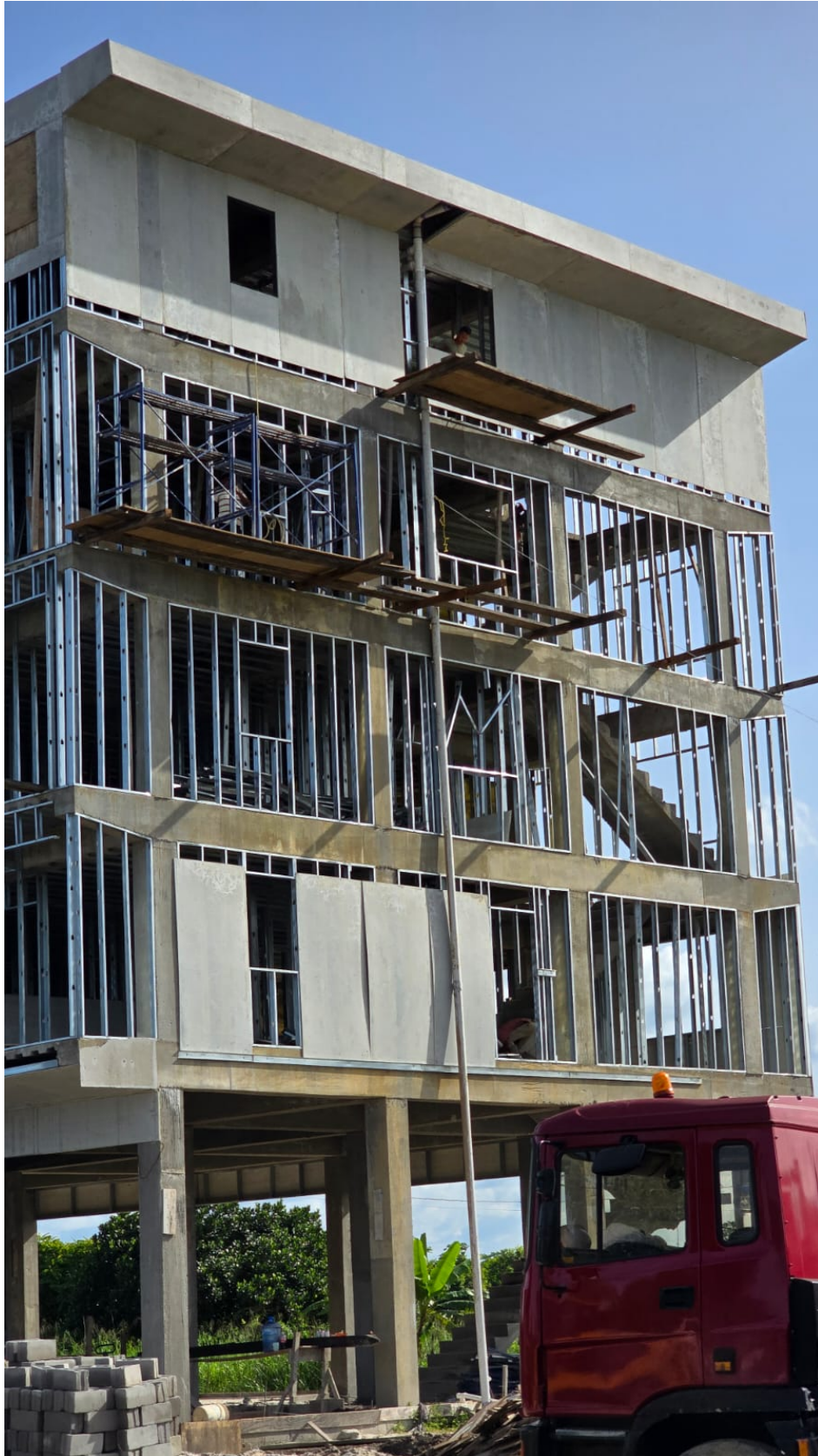
<Figure 15: Unfinished Front of Erected Hotel Building>
