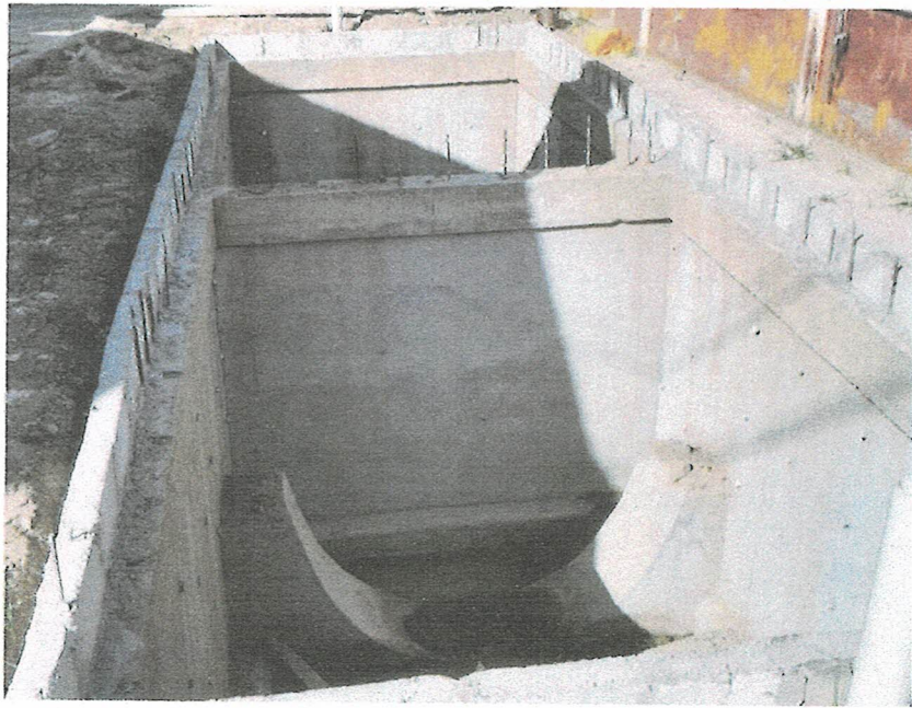
Figure 4. Pictures of reinforced concrete containment (completed)
