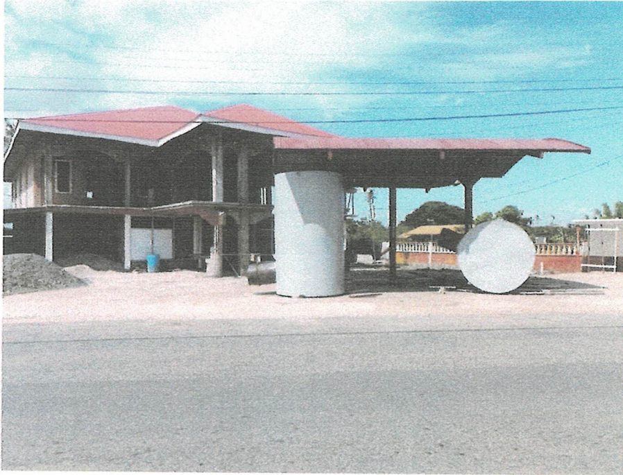
Figure 2. Picture of the service station's canopy and tanks for underground storage
