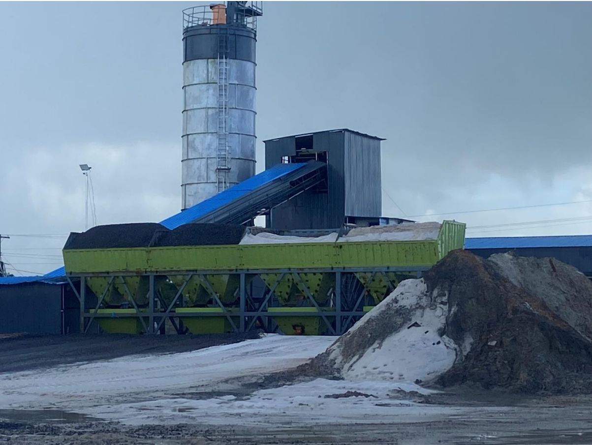
Image 5: Cement Mixing Station
