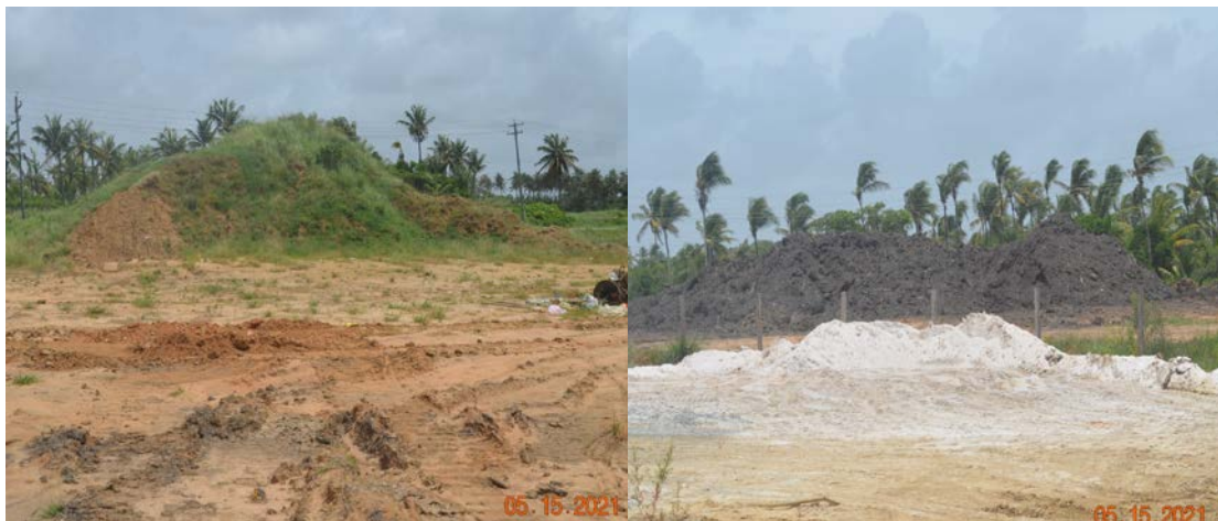
Photo 8: Earthen material stockpiled
