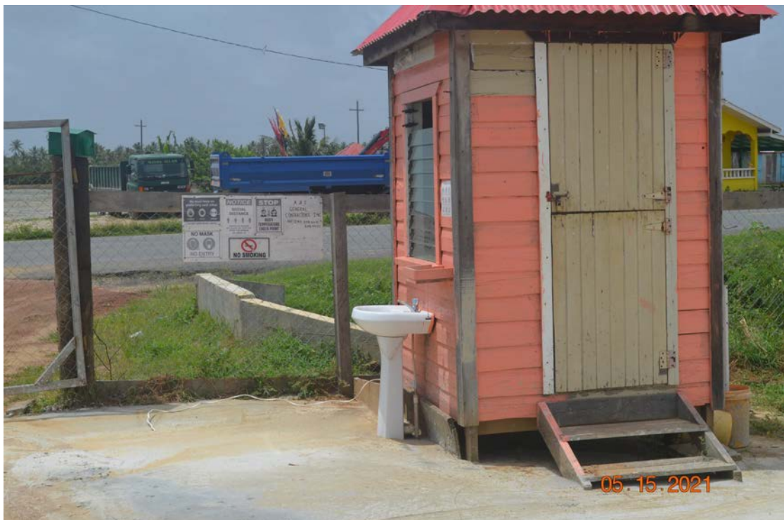
Photo 6: Hand wash Station
