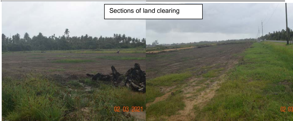
Photo 1: Land clearing at the project site
