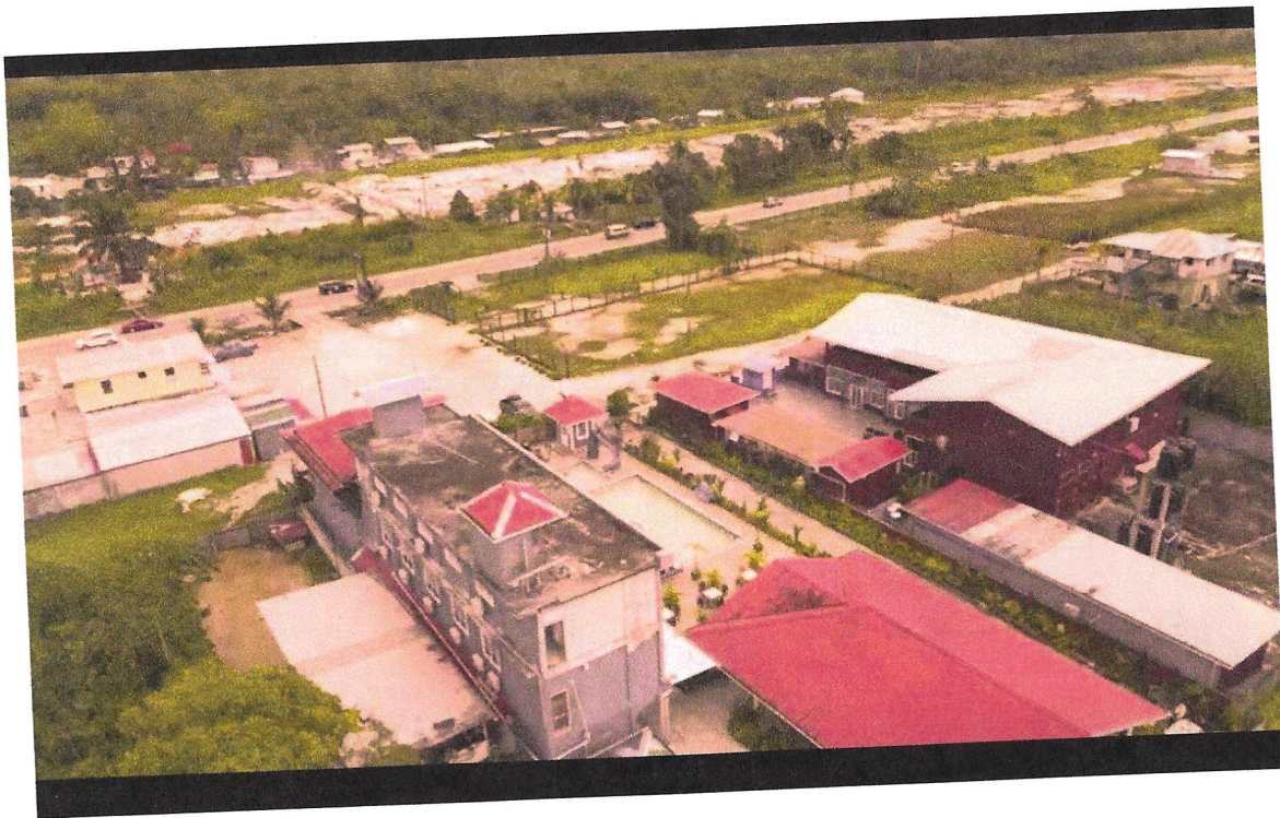
Image 1: Aerial view of activities surrounding the Plasma Rock facility (see section 2.0 for details).
