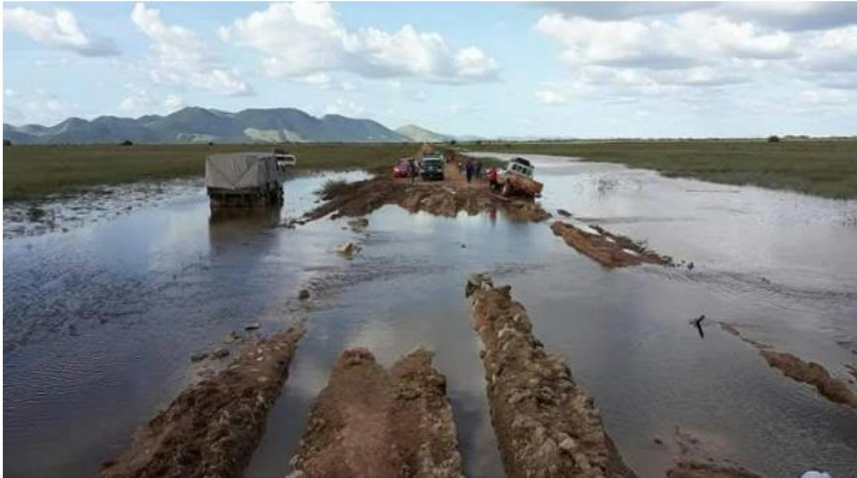
Figure 24: Flood damage to the Lethem-Georgetown Road in July 2017.
