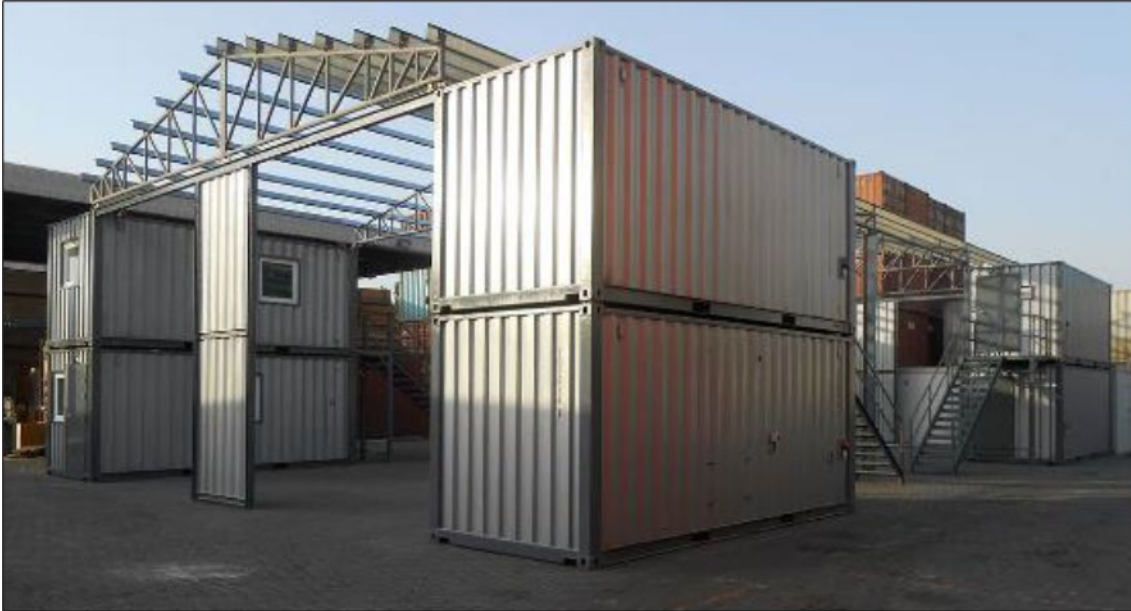
FIGURE 1.4 CONCEPT FOR MOBILE EQUIPMENT MAINTENANCE FACILITY
