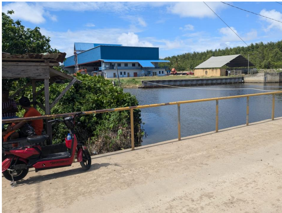
Image 4 Drainage channel for the Lusignan Pump Station.
