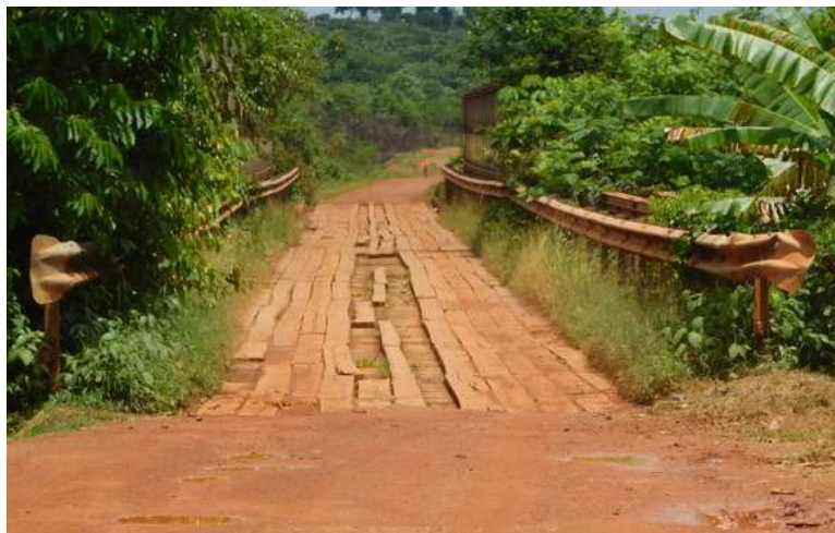
Figure 18-9: Eclipse Falls Bridge
