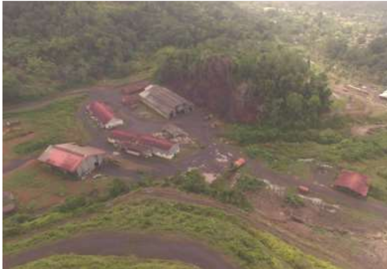
Figure 17-2: Matthew's Ridge Mine Site Infrastructure, August 2018
