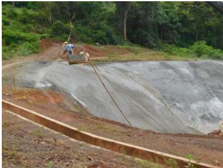
Figure 17-16: Concrete-lined Storm Water Trench and Slope Stabilization
