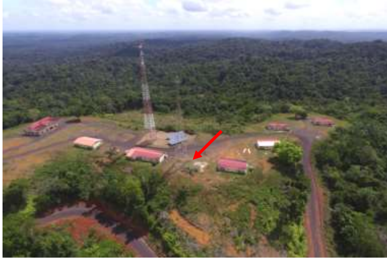
Figure 17-1: Communication Towers, Staff Accommodation Matthew's Ridge (August 2018)
