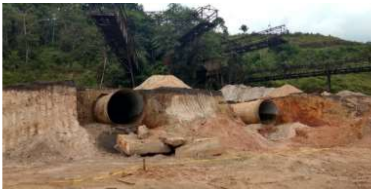
Figure 20-2: Tunnels from which Bat Droppings and Debris were Cleared
