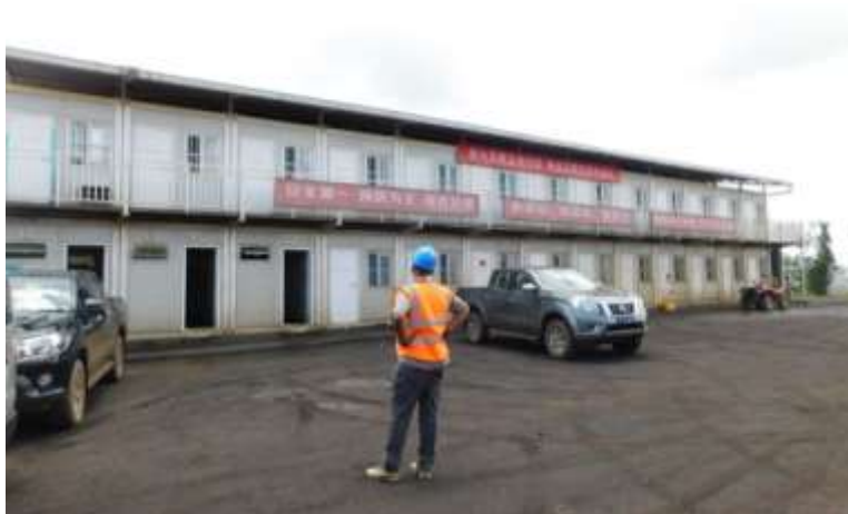
Figure 20-5: Workers Accommodation in Matthew's Ridge
