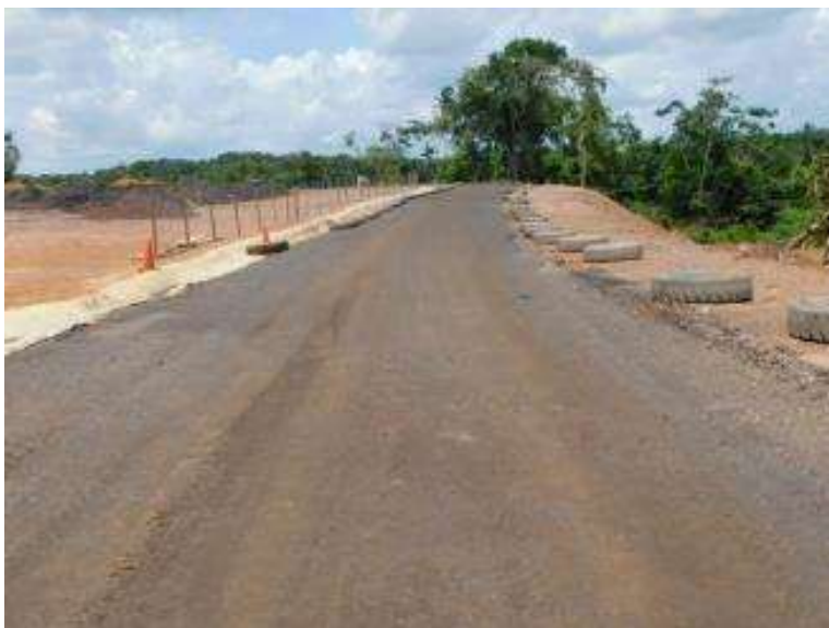
Figure 16-6: Use of Spent Tyres for Road Definition along the Matthew's Ridge Airport Bypass Road
