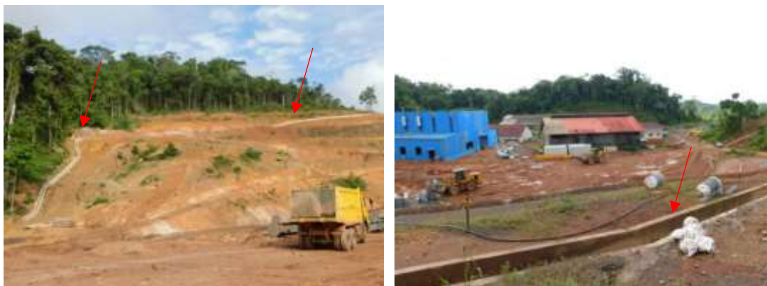
Figure 8-8: Storm Water Drains Constructed by GMI
