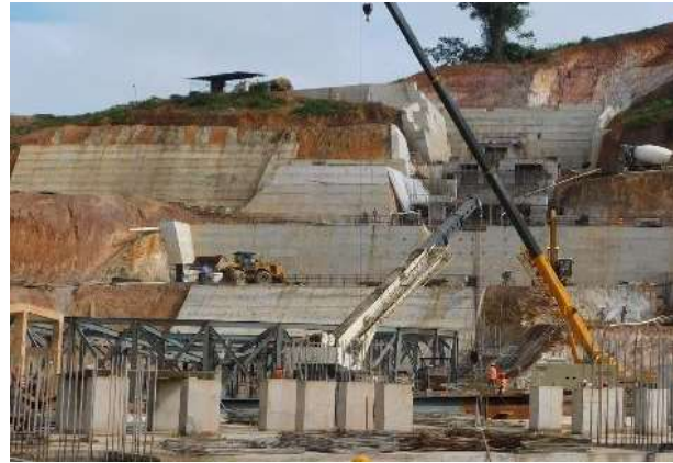
Figure 17-11: Process Plant Construction (April 2020)
