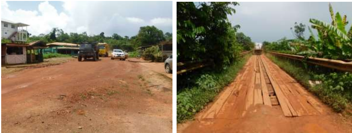
Figure 15-10: Heavy Vehicles passing through the Eclipse Falls Village (left) and on the Eclipse Falls Bridge (right) [July 2020]
