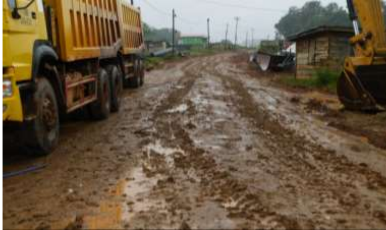
Figure 15-4: Road Leading from the Log Pond Facility (January 2020)
