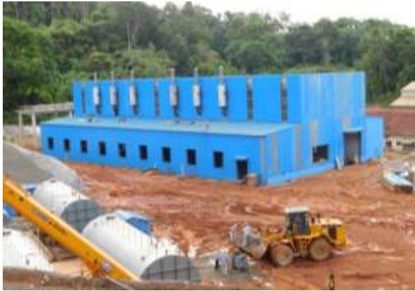
Figure 17-10: Matthew's Ridge Power Plant Reconstruction (July 2020)
