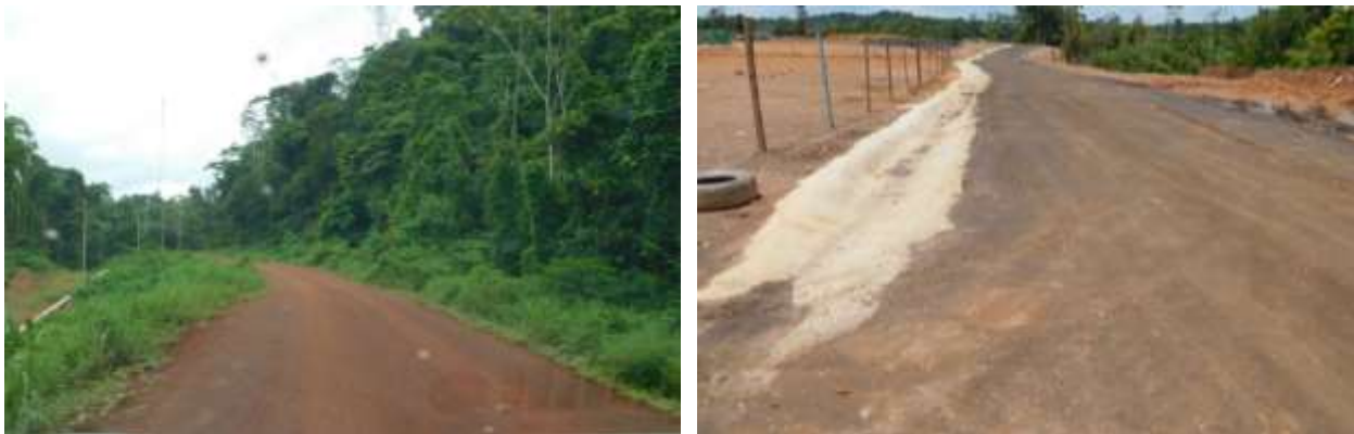
Figure 15-7: Newly Constructed Bypass Road around the Matthew's Ridge Community (left) and around the Processing Plant to the Airstrip (right) [July 2020]
