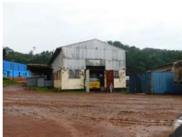
Figure 18-6: Rehabilitation of Previous Mines Buildings
