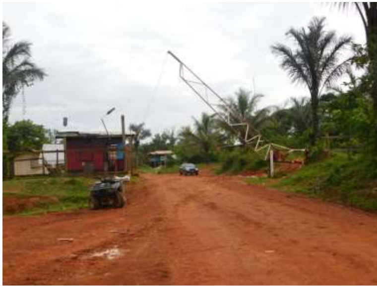
Figure 15-3: NDC Toll Booth at Four Miles
