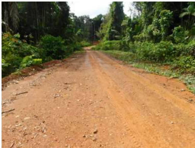
Figure 15-5: A Section of the GMI Bypass Road to the Kaituma Marine Terminal (January 2020)
