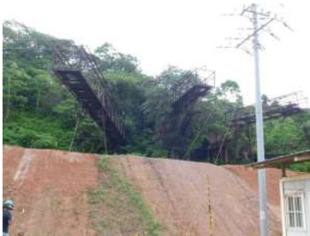
Figure 18-5: Remnants of the Old Processing Facility
