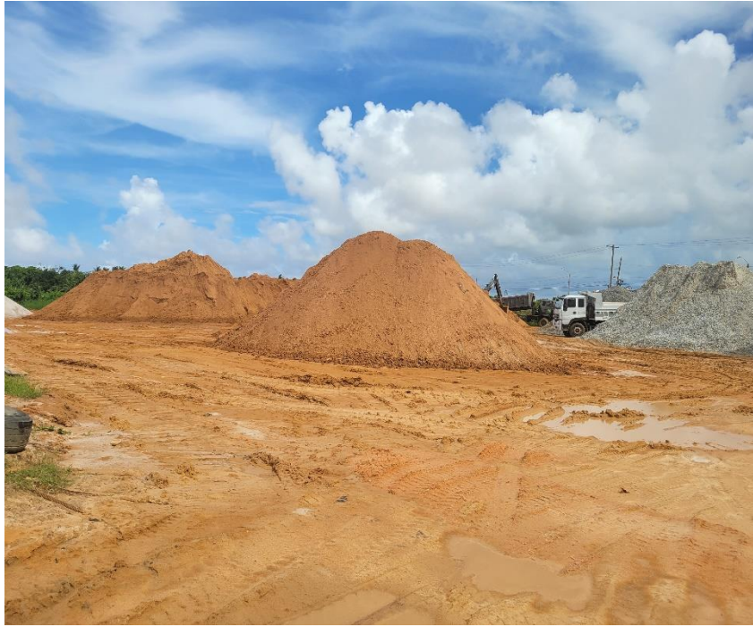
Picture showing a section of the stockpile area at the site.
