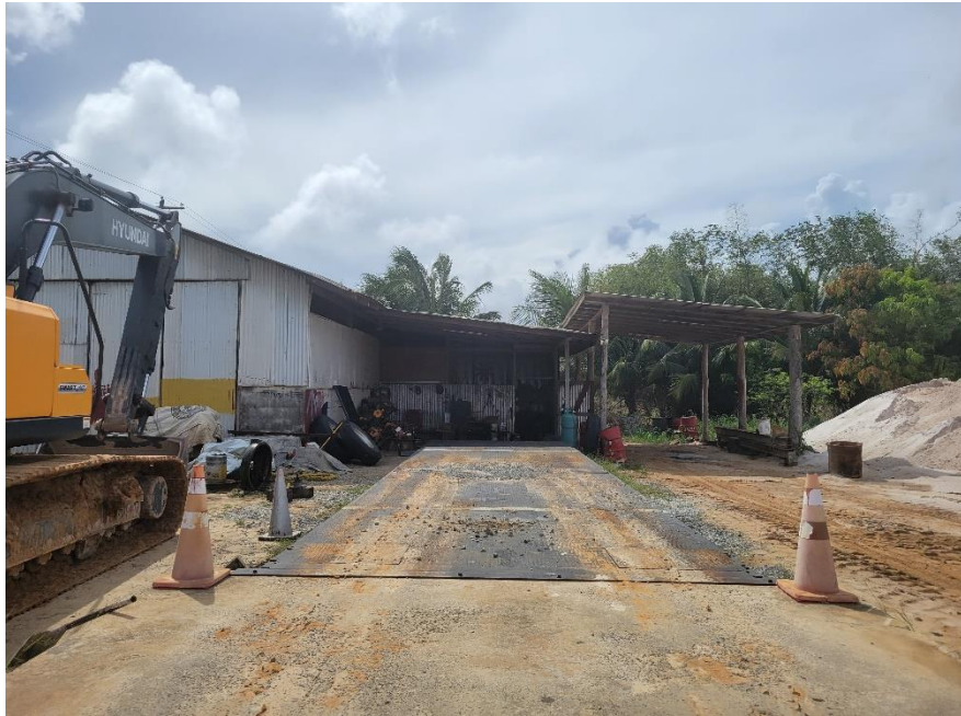
Picture showing the storage shed and minor repair shed at the site.
