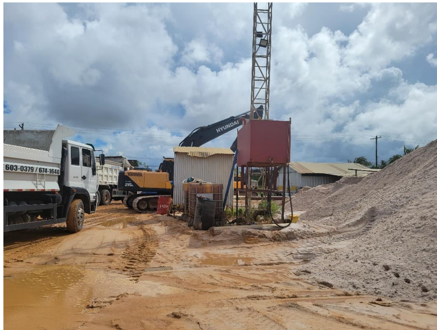
Picture showing the fuel storage area at the site.
