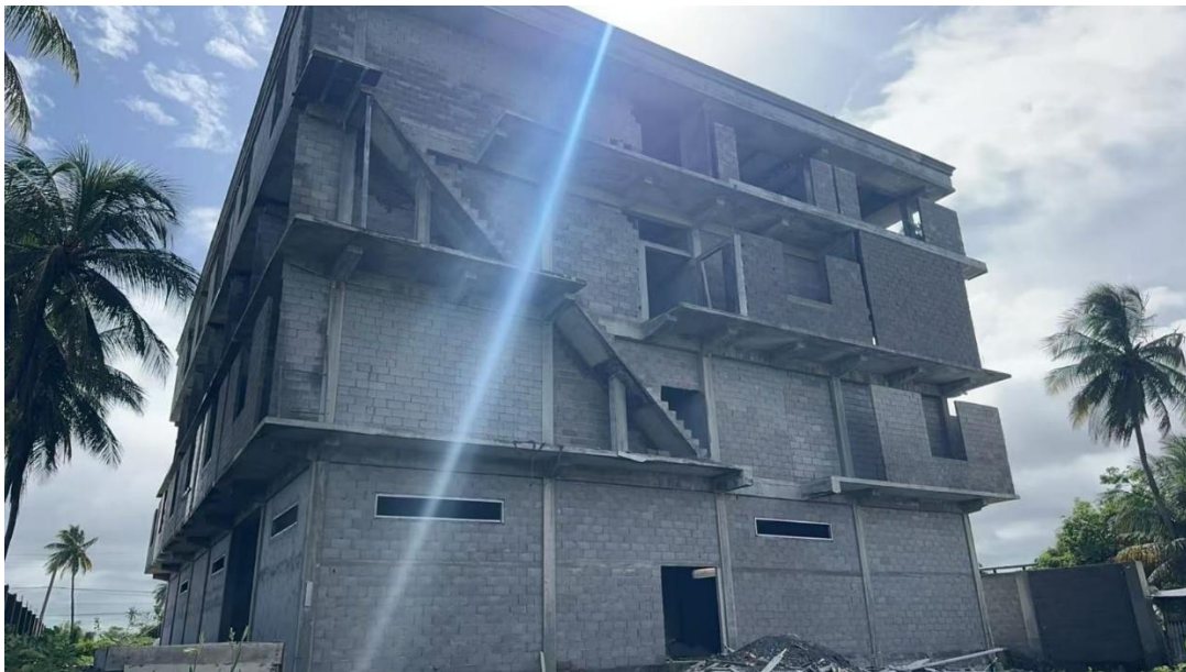
Picture 2: Emergency stairs of the hotel under construction
