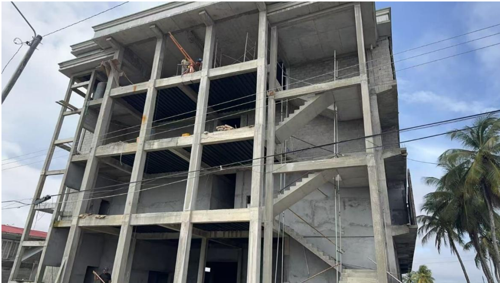
Picture 1: Hotel under construction
