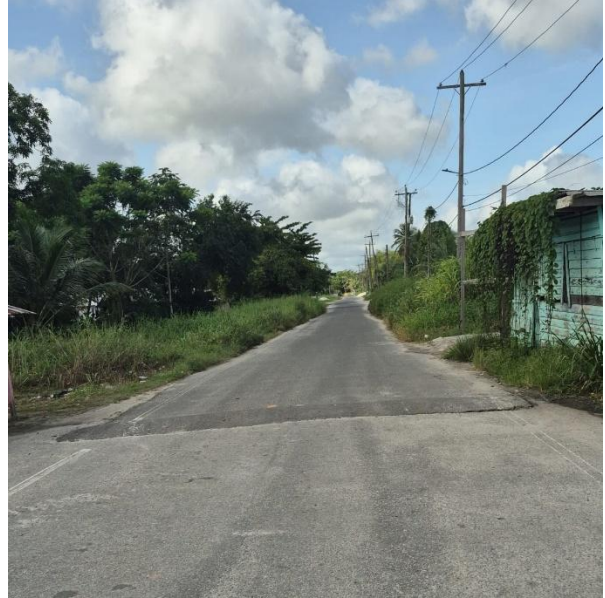
Figure 9: Secondary Asphalt Road
