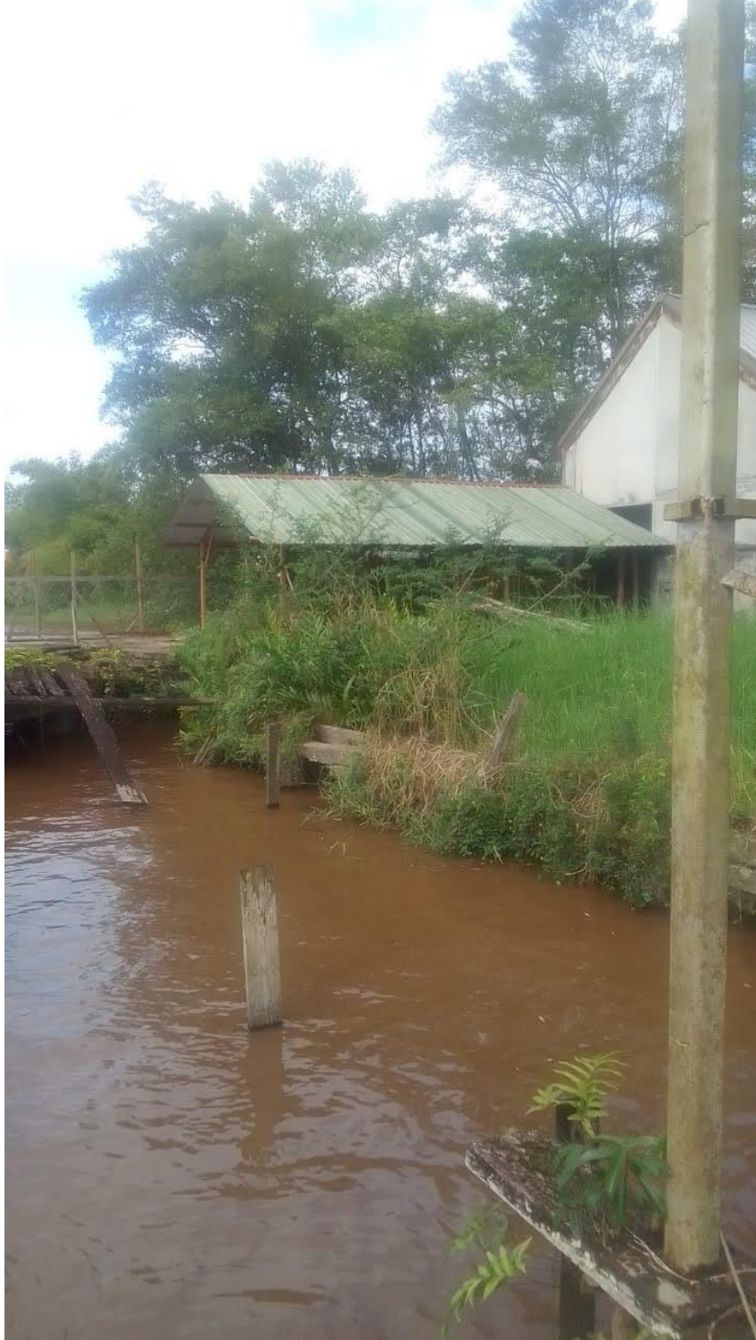
<Figure 5: Fuel Intake/ Outlet Line Point near Wooden Wharf>
