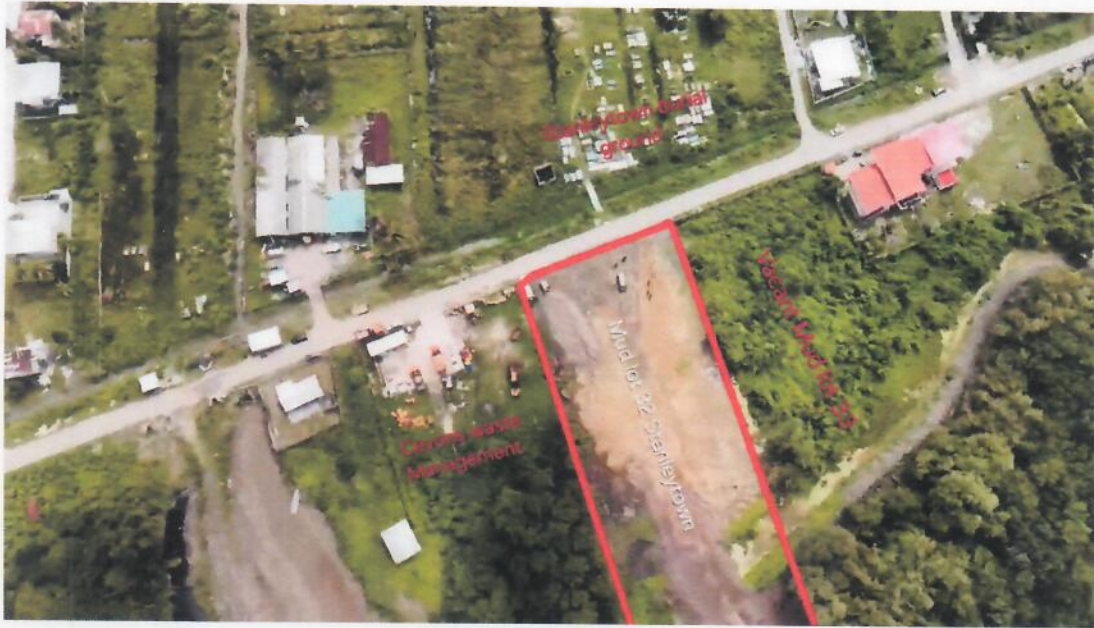
Figure 1 Aerial view of surrounding designated lot for Wharf construction.
