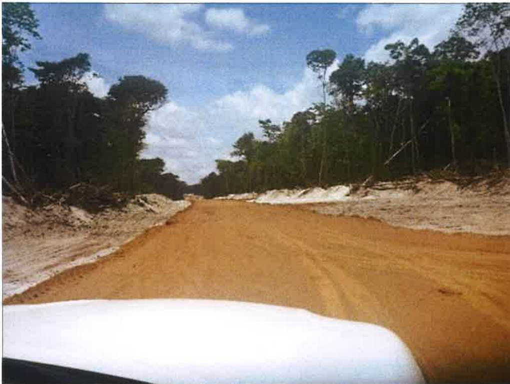
Photo 2: New Thriving and Arisaru North Quarry Project access road.
