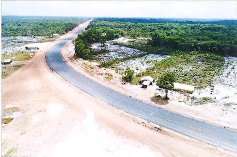
Photo 1: Drone view of Linden-Mabura asphalt road under construction.
