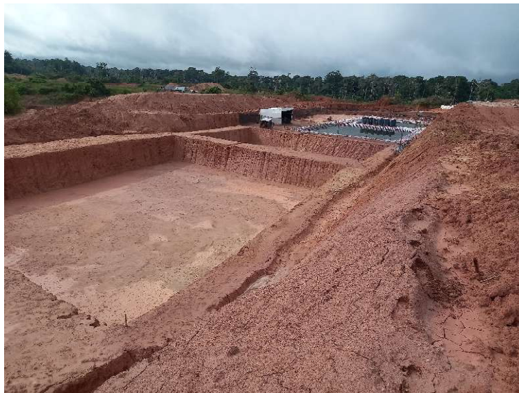
Figure 6: Heap Leach Facility under Construction.
