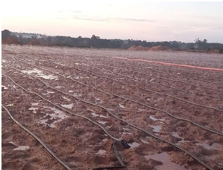
Figure 7: Lixiviant be added to a Stacked Leach Pad.
